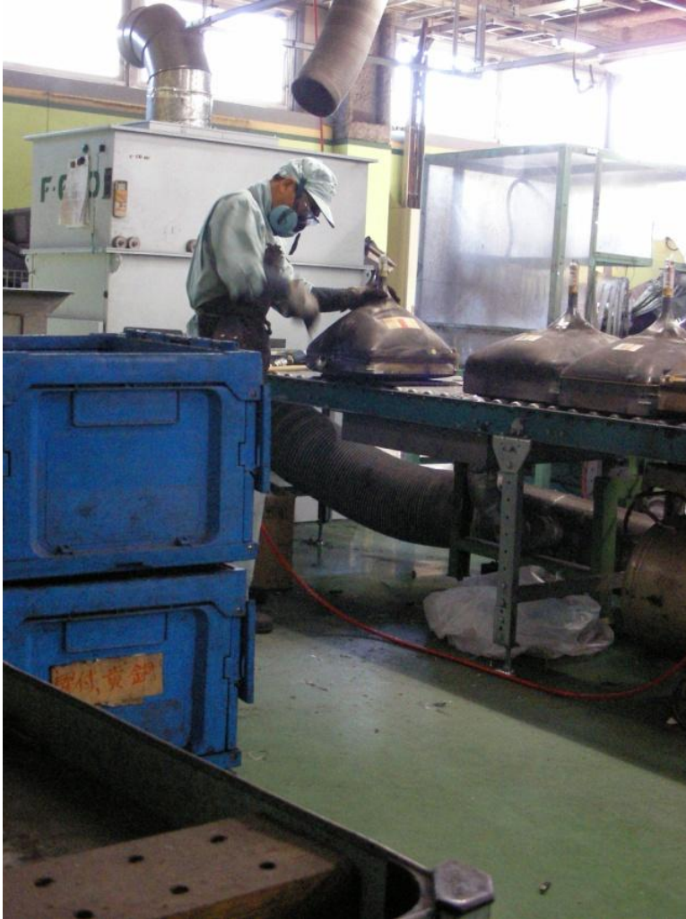
Dust collection is installed in home appliance dismantling facility in Tokyo, Japan, 2007.
