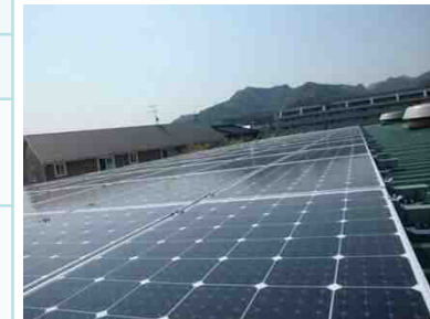
Solar power generation system
