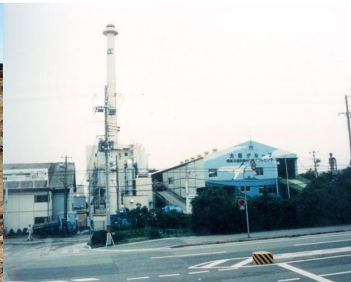
1984 Daiei Kankyo Nishinomiya Branch started business (City of Nishinomiya, Hyogo Prefecture)
