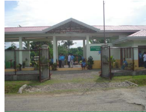
Materials Recovery Facility
