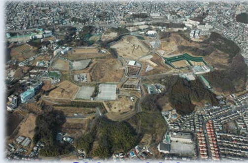
Shinmeidai Final Disposal Site
