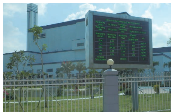
WtE Plant at Thoi Lai
