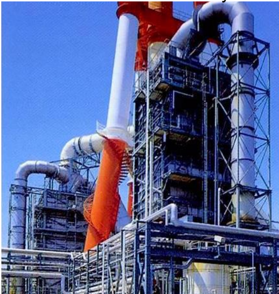
Exhaust gas desulfurization facility
